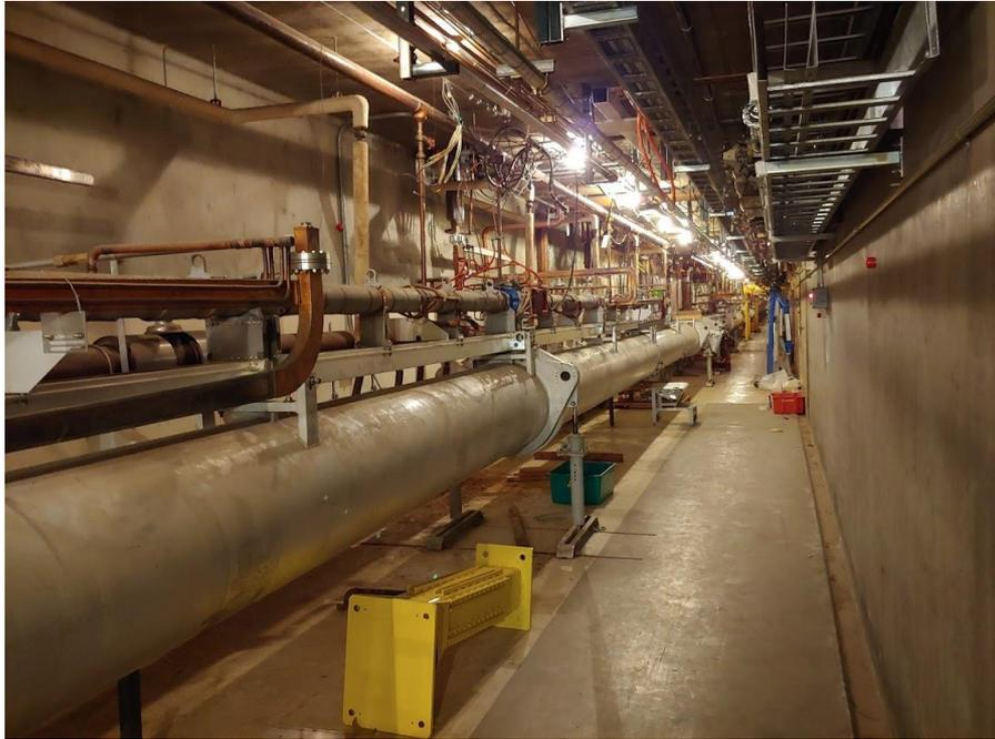
Large pipe is laser tube with Fresnel Lens for alignment as a strong back.
